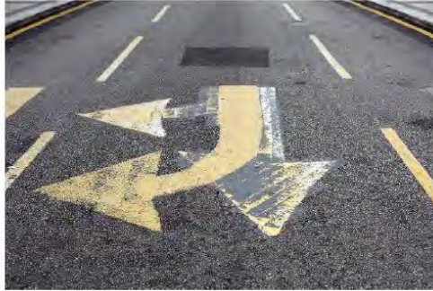
Figure 3-2. Example of overlapping pavement markings
