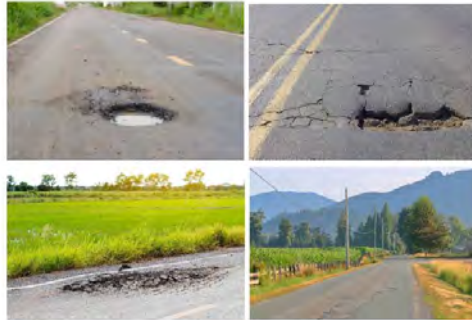
Shutterstock Figure 3-9. Examples of road surface degradation
