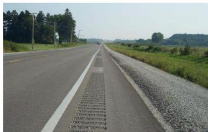
Shoulder Rumble Strips
