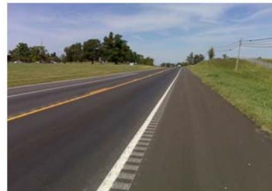
Edgeline Rumble Strips
